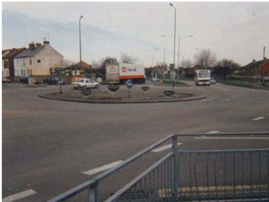
Figure 1. Gloucester 'Before' Roundabout Modifications
