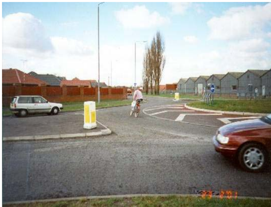
Figure 3. Nottingham 'After' Demonstrating Larger Central Island
